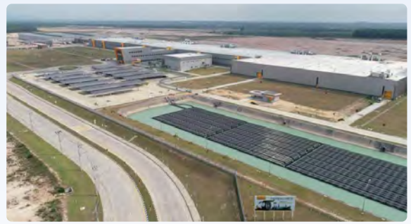
Floating Solar System
